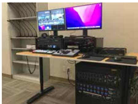
Finished MYPA Install
